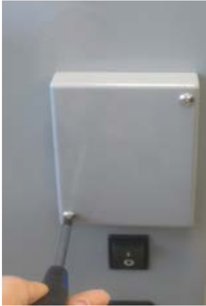
Figure 4: Controller Cover Removal
