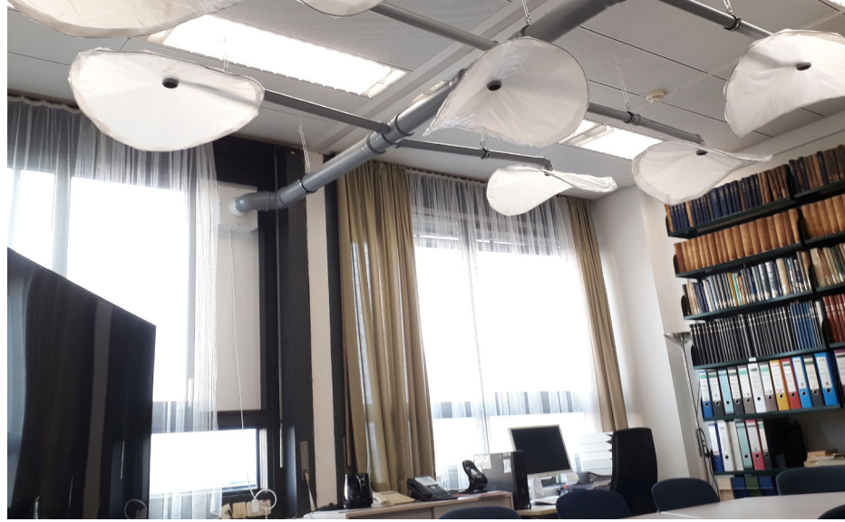
Fig. 2: Installed ventilation system with extractor hoods.
